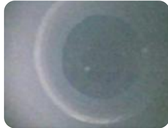
Filter recirculation pipe 22 days after mixed oxidants
